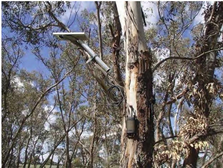
Photo 9: SPPM used on the branch of a tree.
